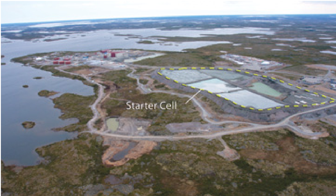
Photo above: Aerial view of the North Pile
